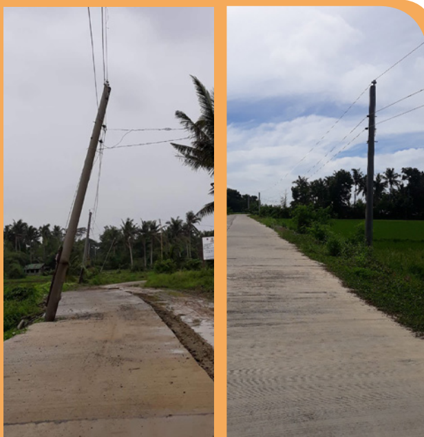
BEFORE and AFTER photos of relocated electrical poles at Malekkeg, Sta Marcela in Apayao to construct national government's project of road concreting.
