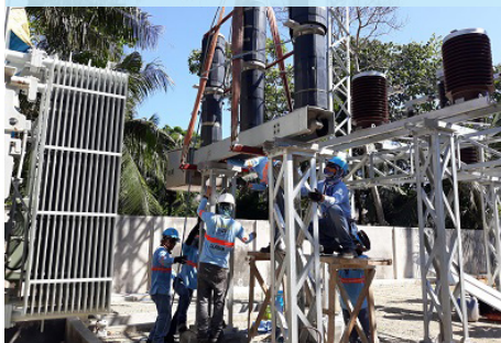
Construction of the 5/6.25 MVA Sanchez Mira Substation
